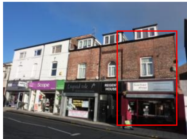
Photograph 12: No. 10 Regent Road
