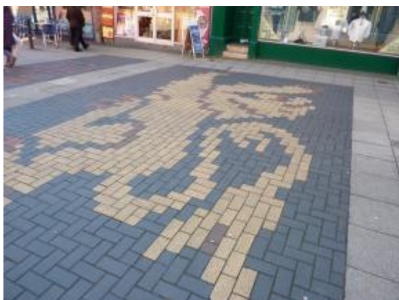
Photograph 15: Brickwork on Cross Street
