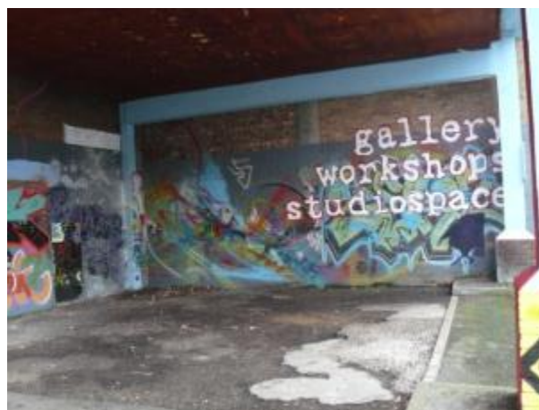
Photograph 25: Space Underneath the Intrusive Structure to Rear of 72 George Street
