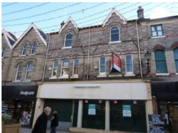
Photograph 13: Vacant shop with intrusive 'to let' board.
