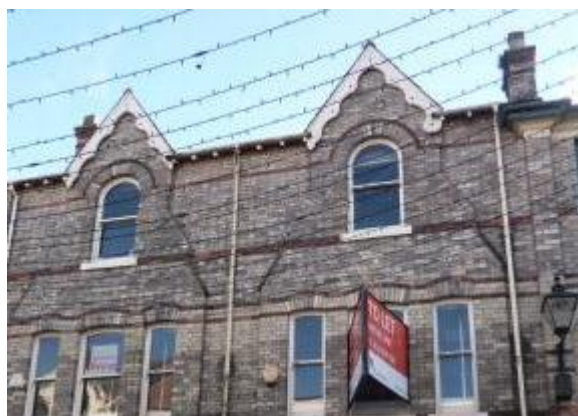
Photograph 18: Decorative Barge Boards
