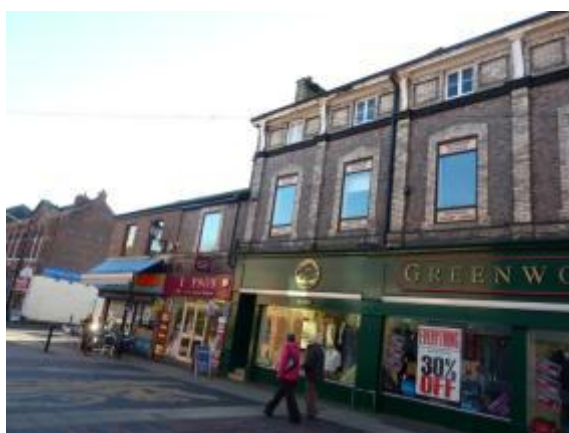
Photograph 7: 69 George Street, an example of classical revival with polychromatic brick pilasters and façade divided into classical proportions
