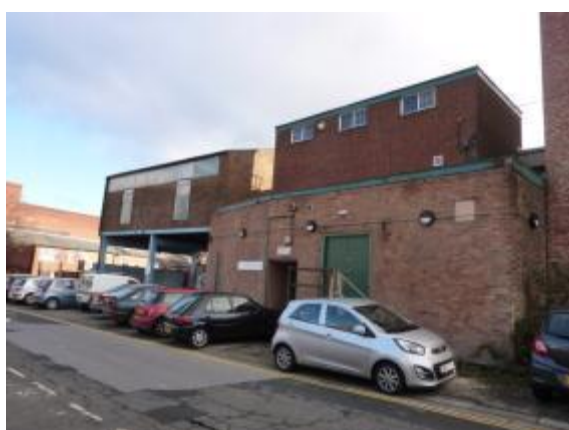
Photograph 22: Mid to late 20 th Century Building on Central Way
