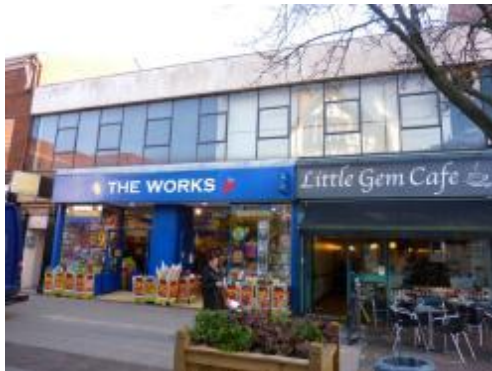
Photograph 9: Inappropriate Signage, No. 77
